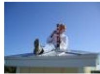
**Figure 2: Using level to make sure rod is plumb**
