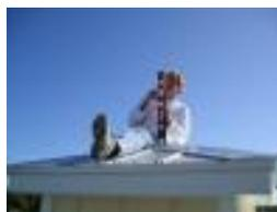
**Figure 2: Using level to make sure rod is plumb**
