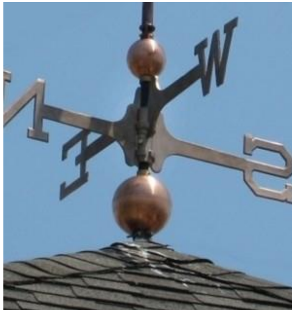
Incorrect Harness Assembly & Placement Directionals are not interlocked
